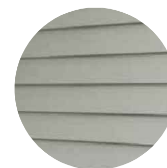
Upper Walls - Weatherboarding
