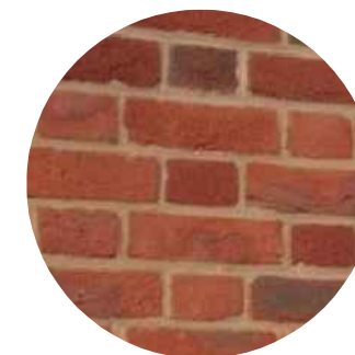
Lower Walls - Brickwork
