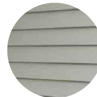
Upper Walls - Weatherboarding
