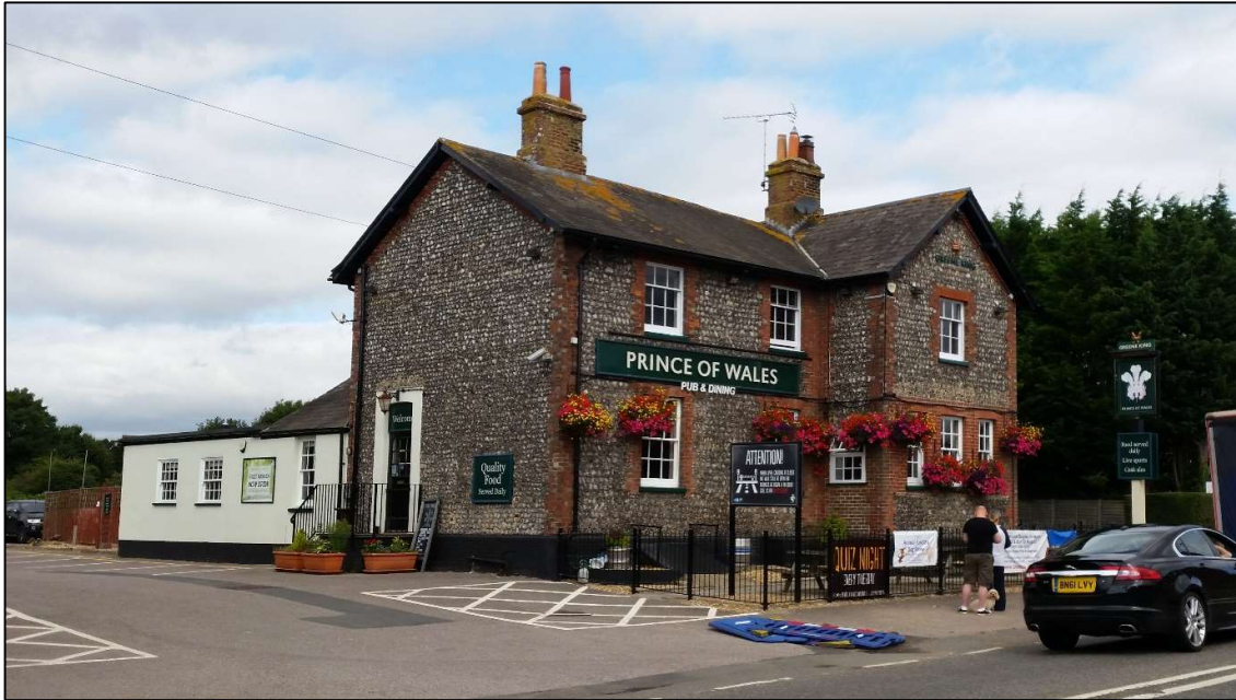
Prince of Wales Public House, 200m to the north of the application site.
