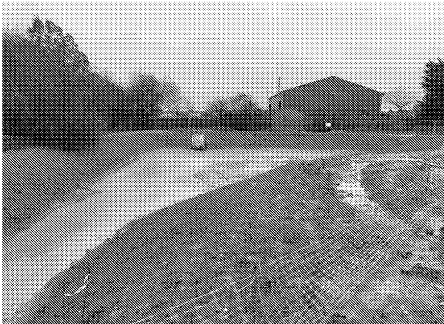
Attenuation Basin Following Construction.
