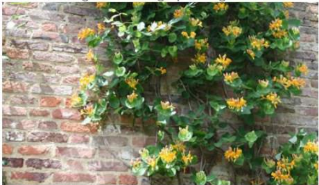
Climbers to substation on support trellis
