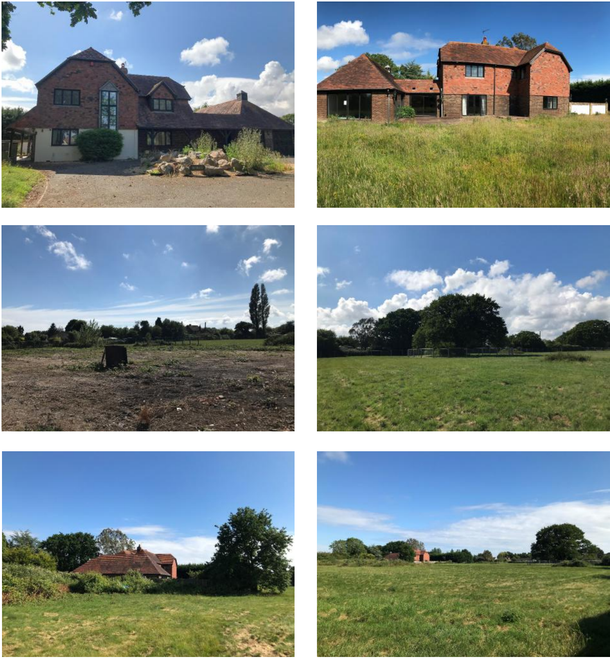
Images of the site and existing building
