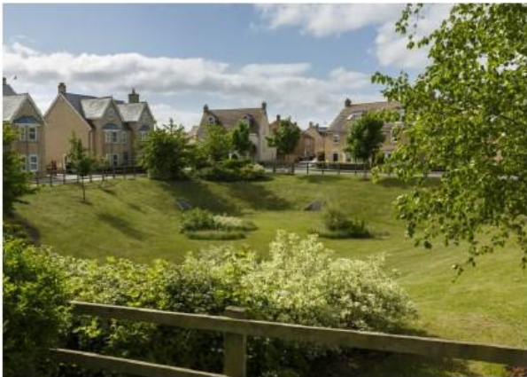
Dry attenuation basin
