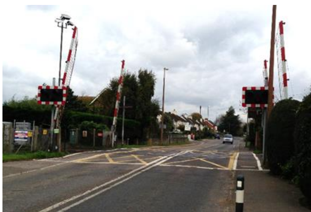
Woodgate Level Crossing
