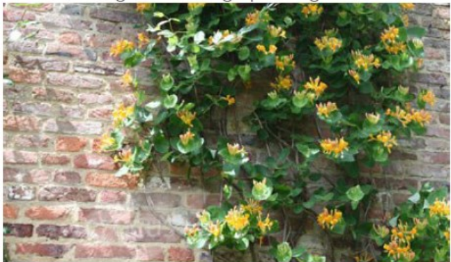
Climbers to substation on support trellis
