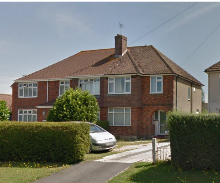
Local precedence, semi-detached brick and tile hanging on Lidsey Road
