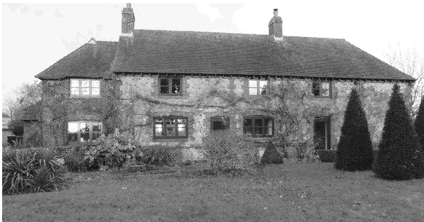
Photograph No. 1 - View of the south-western aspect of Building B1. - The Old Cottage
