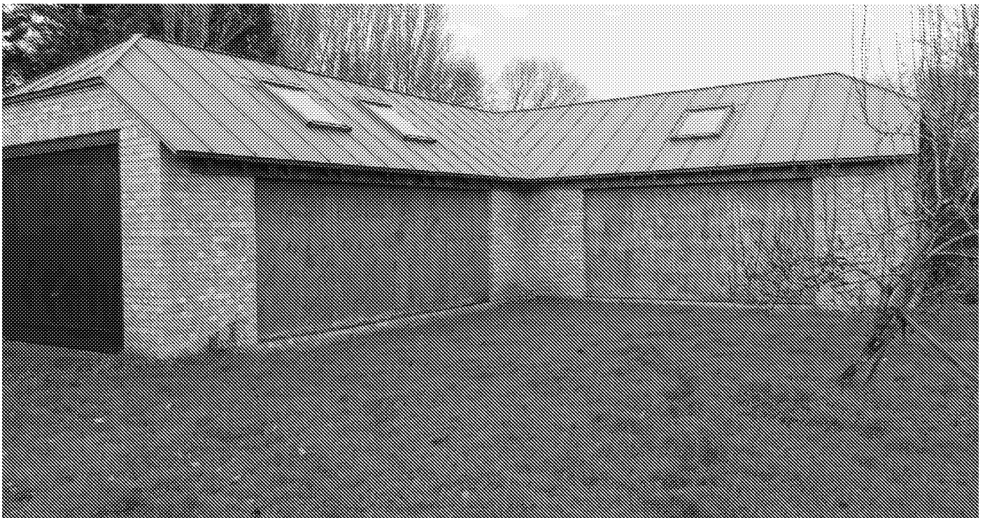
Photograph No. 6 - Building B3, assessed as providing 'negligible' bat roost suitability. - The Old Cottage.
