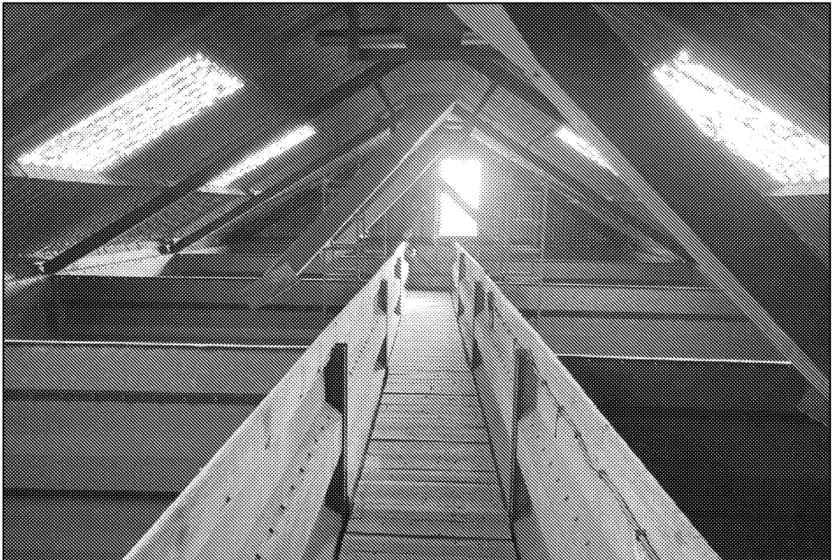
Photograph 3. The raised walkway between large metal grain hoppers within the upper level of Building B.
