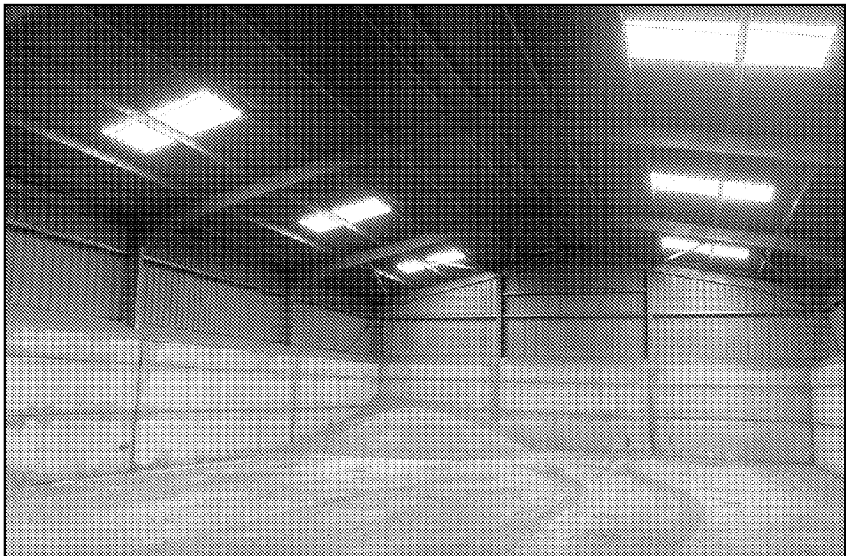
Photograph 5. The interior of Building C.
