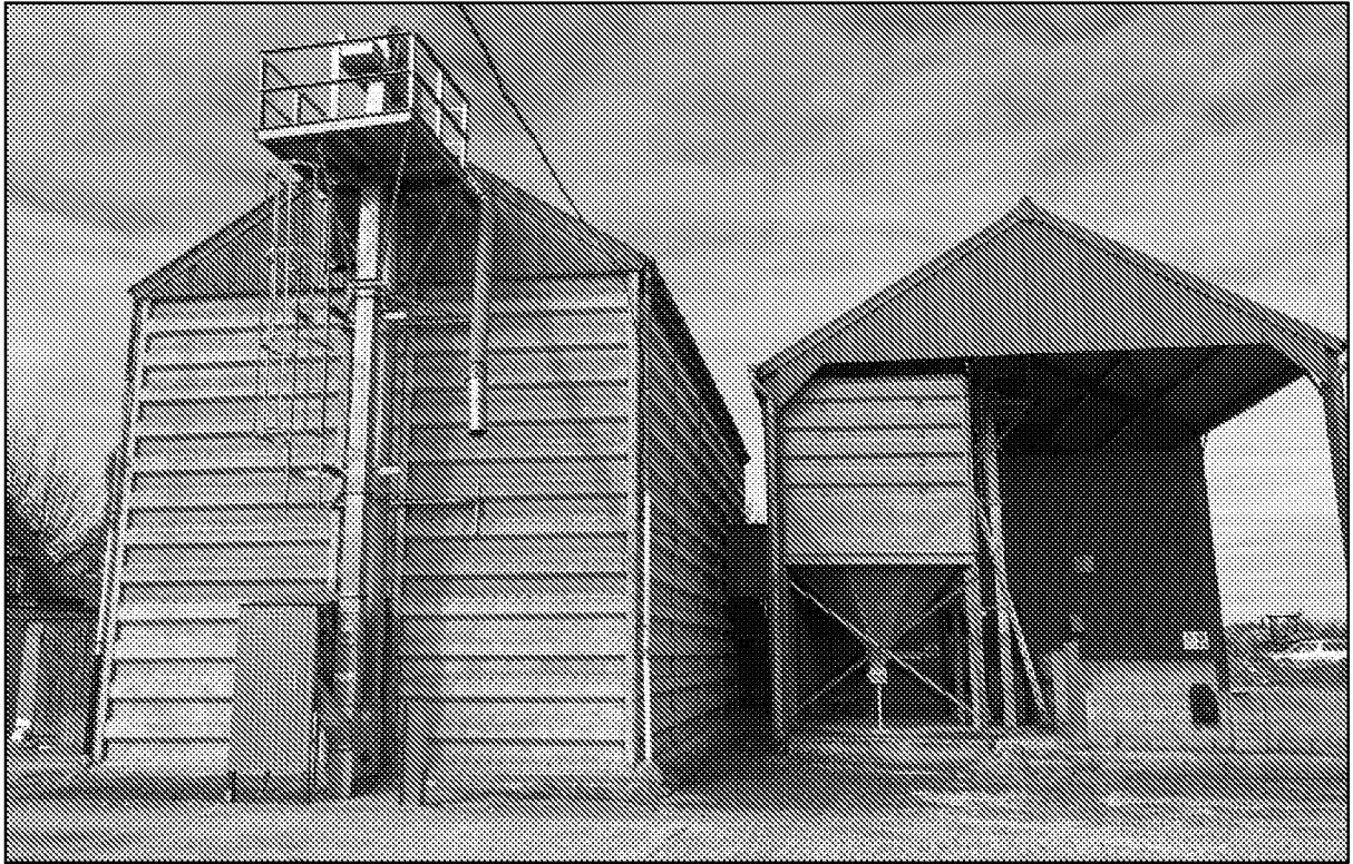
Photograph 2. Building A (right) and Building B (left) viewed from the west.
