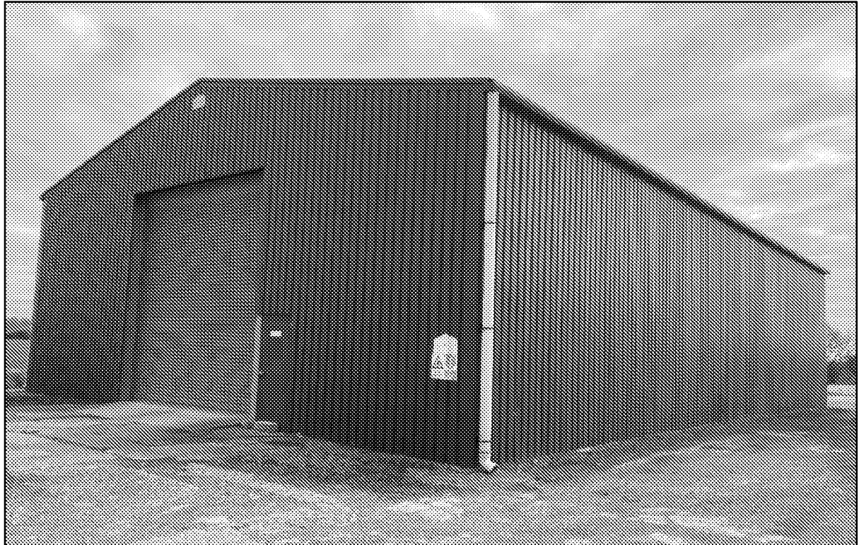
Photograph 4. Building C viewed from the south-west.
