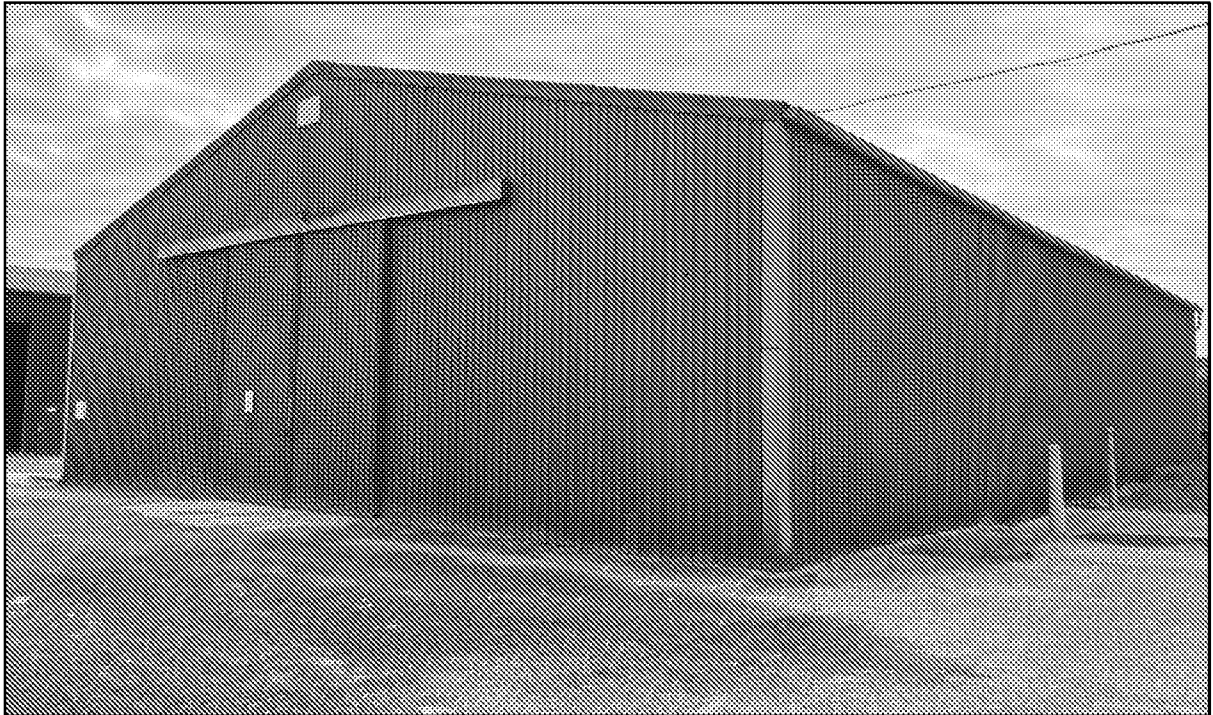
Photograph 6. Building D viewed from the north-west.
