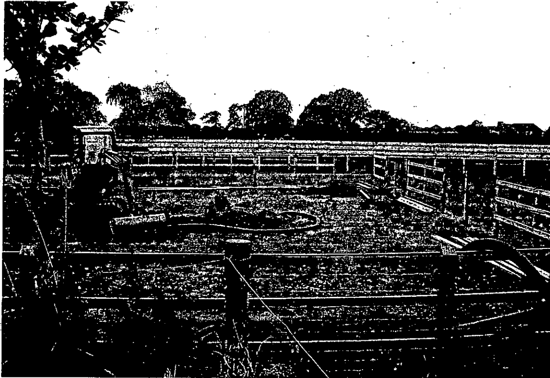
NEIGHBOURS — CONSTRUCTION MENAGE AL/85/08 SEPT 2007 PHOTO TAKEN FROM PROPOSED DEVELOPMENT SITE (pipe trailing onto an property)
