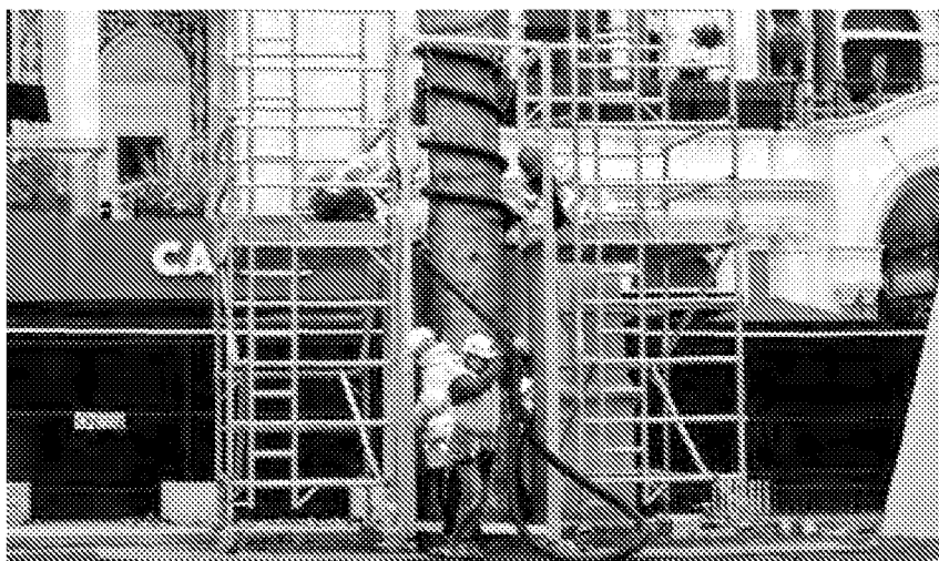
SGN 2-06 Improved use of drainage pipe wrapped around the trunk can provide an added layer of protection beneath a layer of plywood.
