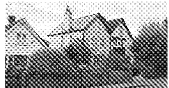
The occasional use of gable elevations (here in a pair, and one of the few three-storey dwellings) provide local focus
