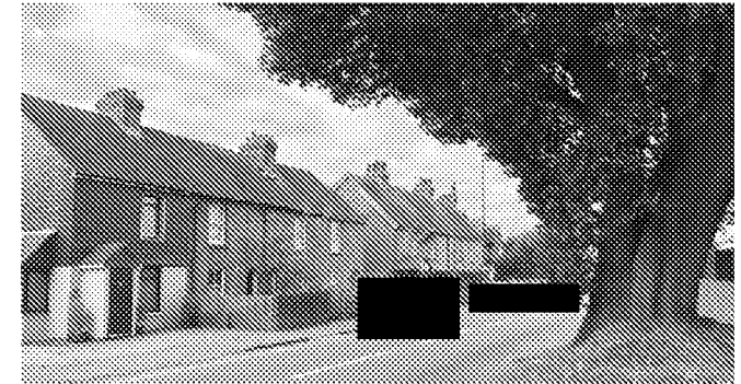
Simple, short eaves-fronted brick terraces between Woodgate and Westergate generally without on-plot parking
