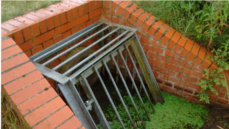
Figure 1-Culvert with Wingwalls and Trash Screen
