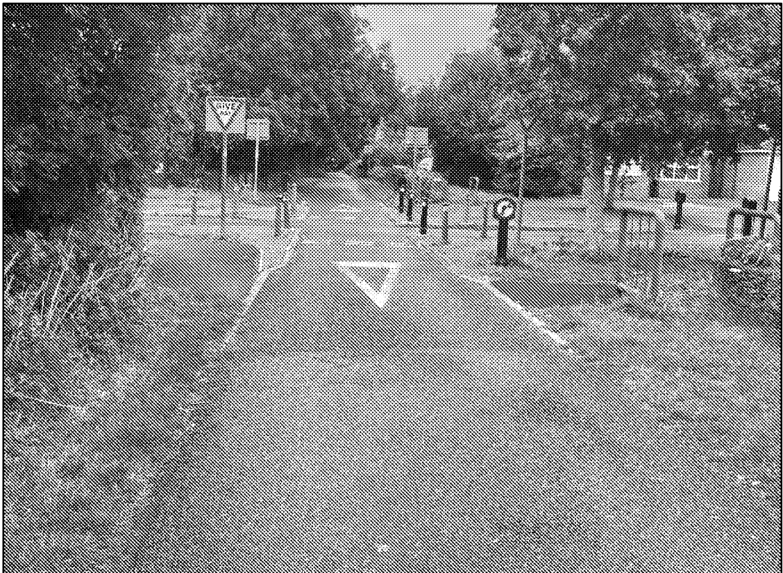
Photograph 4.2 – Example of ahead only crossroad treatment – minor arm
