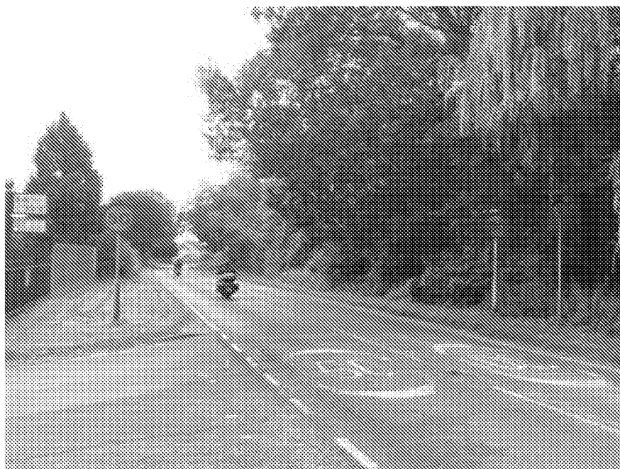
View looking south on A29. The proposed access will be on the right, past the furthest motorcycle
