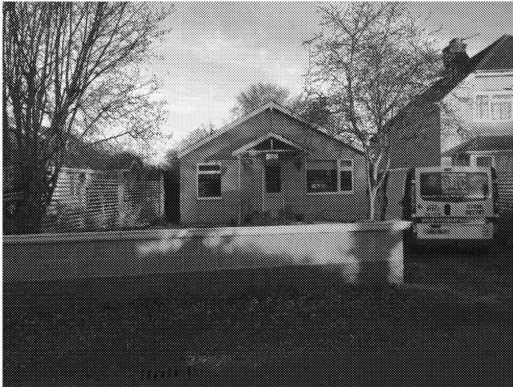
FIGURE 1: Photographs highlighting application site in its current condition
