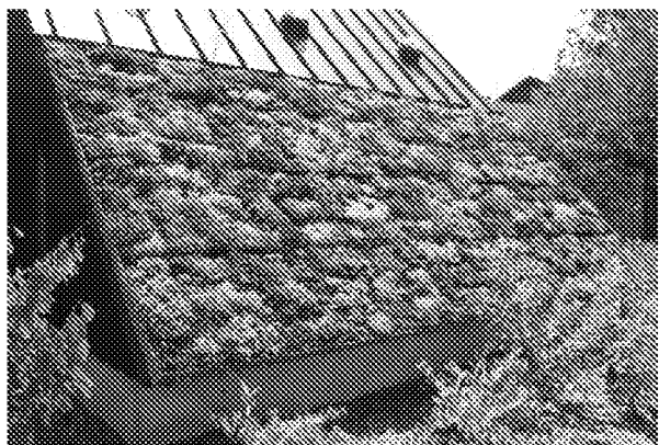
Example extensive, non-irrigated green-roof
