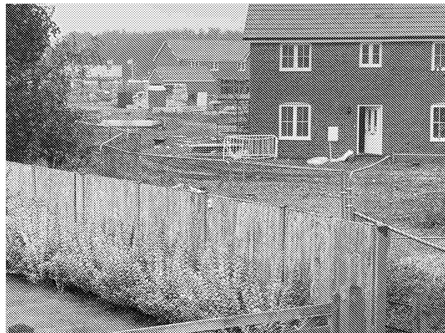
Views of the new residential development adjacent from the site access showing gate
