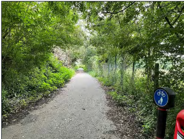
Photograph 8 – Ivy Lane to Church Lane Shared Use Path Eastern End
