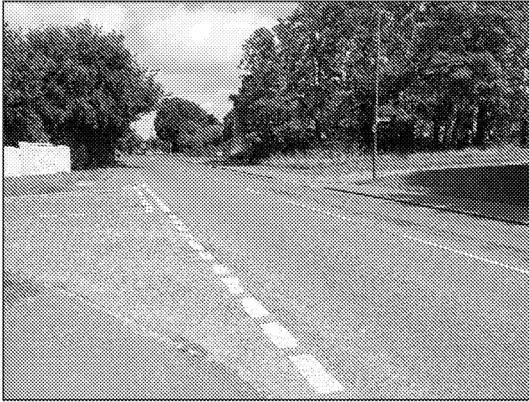
Photograph 1. Existing Site Access and Meadow Way
