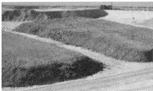
Clearly defined stockpiling of different soil materials
