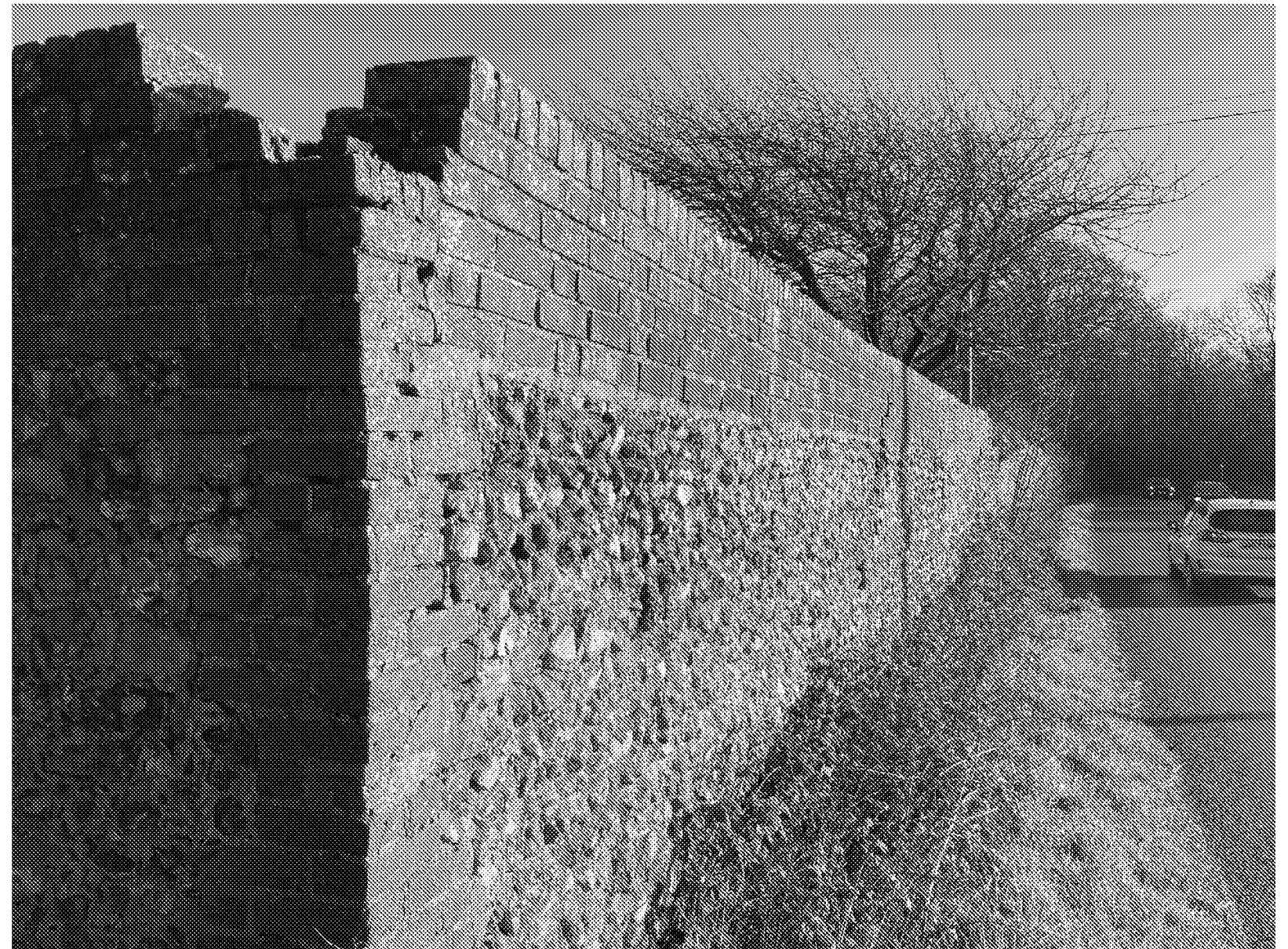
03 Existing Nyton House Boundary Wall
