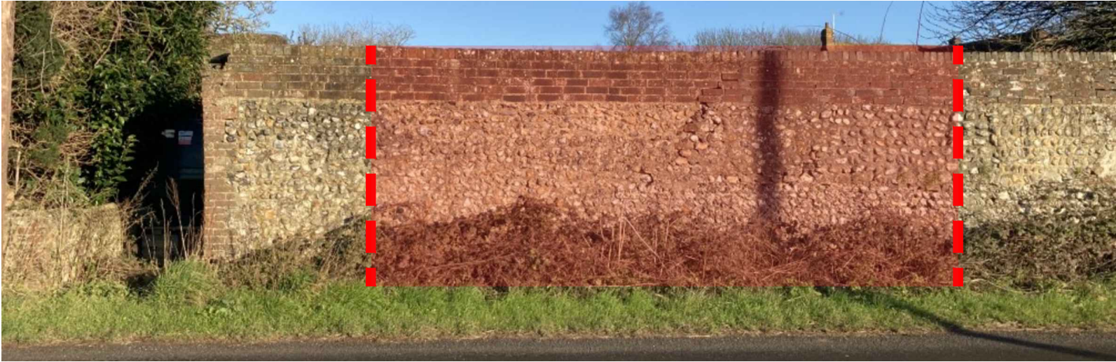
The southern face of the existing wall, as seen from Nyton Road, demonstrating the approximate area to be removed
