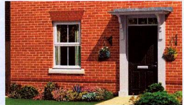
Typical stretcher bond brickwork with contrasting string course & head detail.
