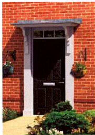
Typical door with GRP surround & gallows brackets.
