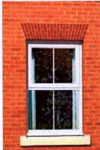
Typical Window style 2
