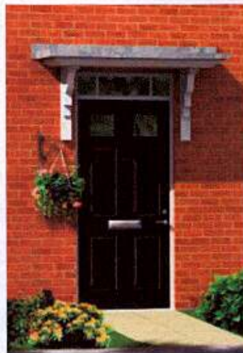
Typical door with flat canopy.
