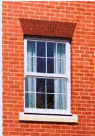
Typical Window style 1
