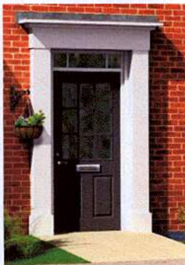
Typical door with GRP surround.
