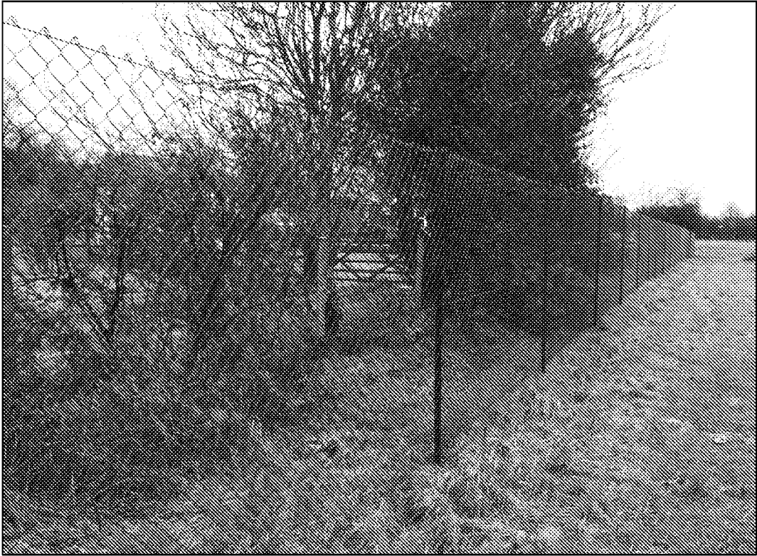
Chain-link on angle-iron uprights
