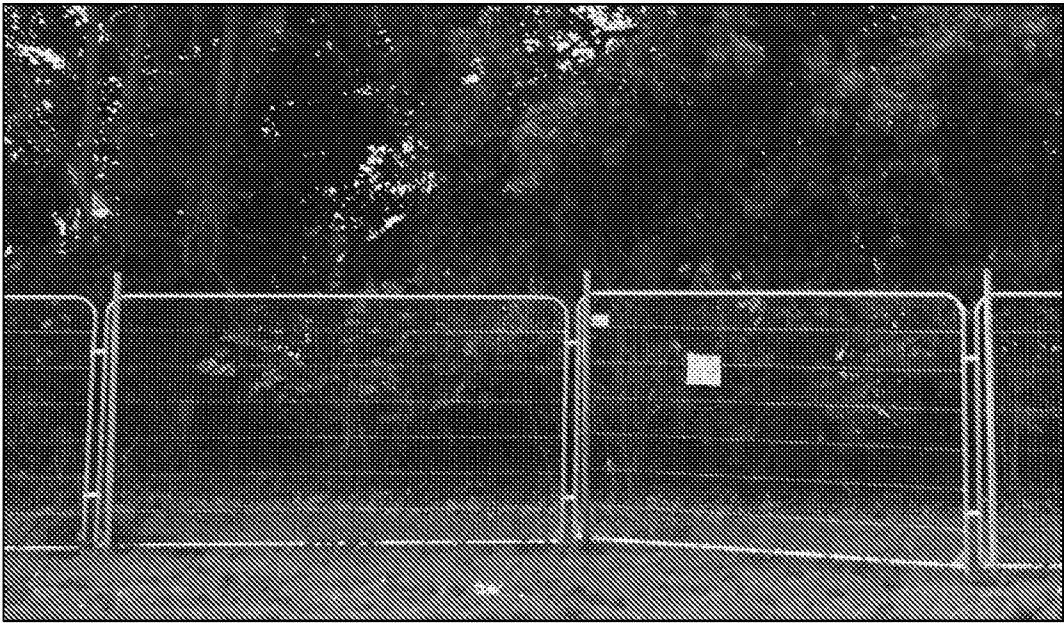
Weld-mesh panels on scaffold uprights
