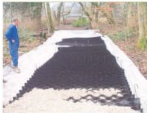
CellWeb during installation.
