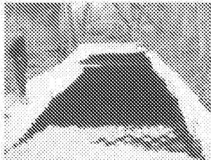
CellWeb during installation.
