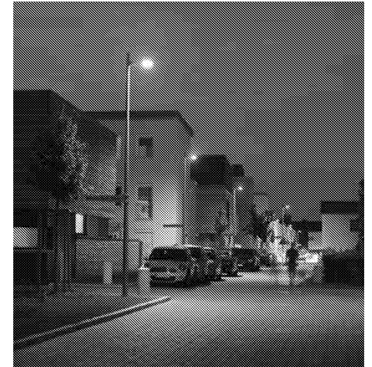
Above: WE-EF LED street & area lighting Below: PV powered LED lights
