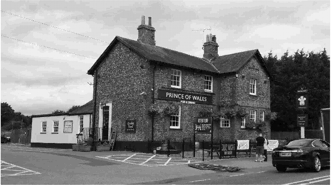
Prince of Wales pub, adjacent to the northeast corner of the site
