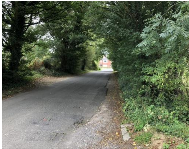
Photograph 1: Conditions on Level Mare Lane
