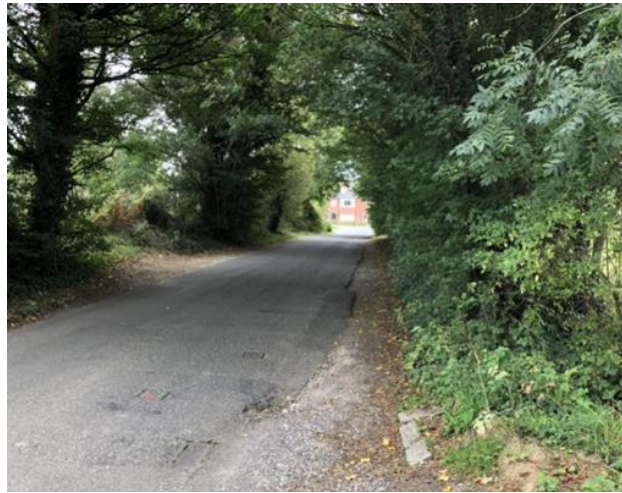
Photograph 1: Conditions on Level Mare Lane
