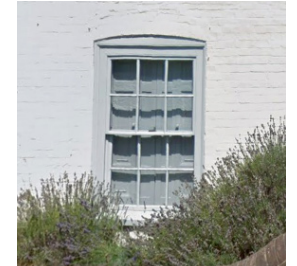
Painted window frames
