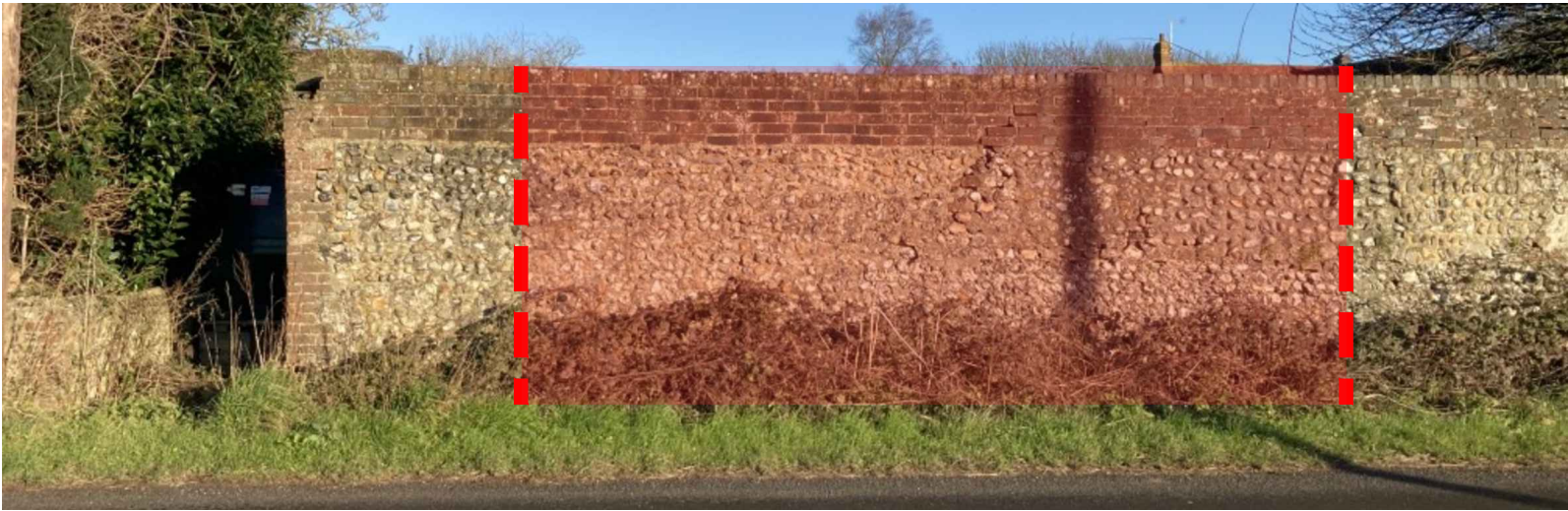
The southern face of the existing wall, as seen from Nyton Road, demonstrating the approximate area to be removed
