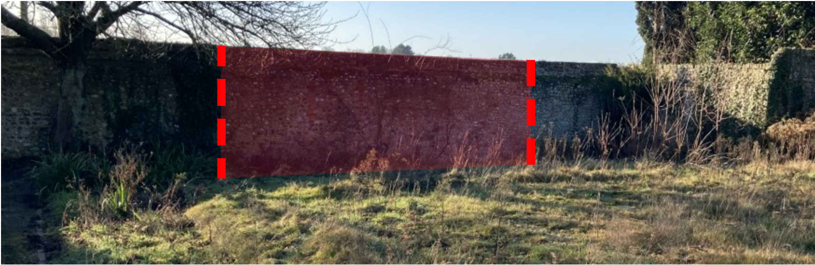
The northern face of the existing wall, as seen from the garden, demonstrating the approximate area to be removed
