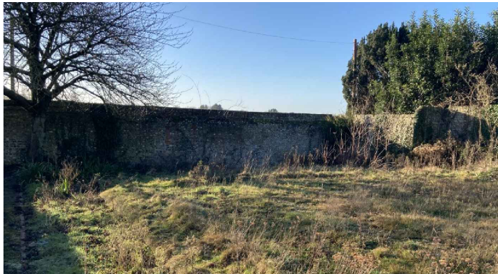
Photo 4 - The extent of the wall as seen from the garden, looking south
