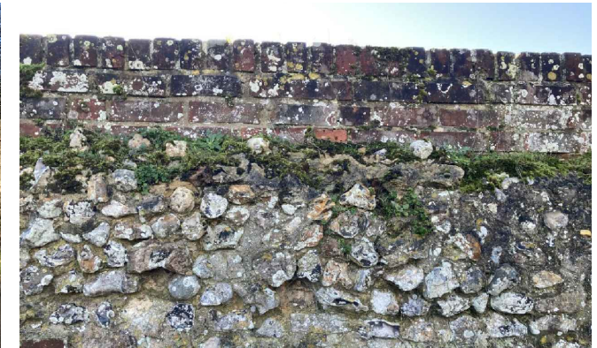
Photo 6 - Close-up of the northern face of wall (as seen from the garden) demonstrating the step of stonework to brickwork capping
