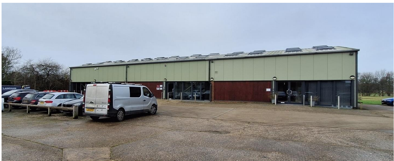
Above: Existing commercial building of West Barn on the site
