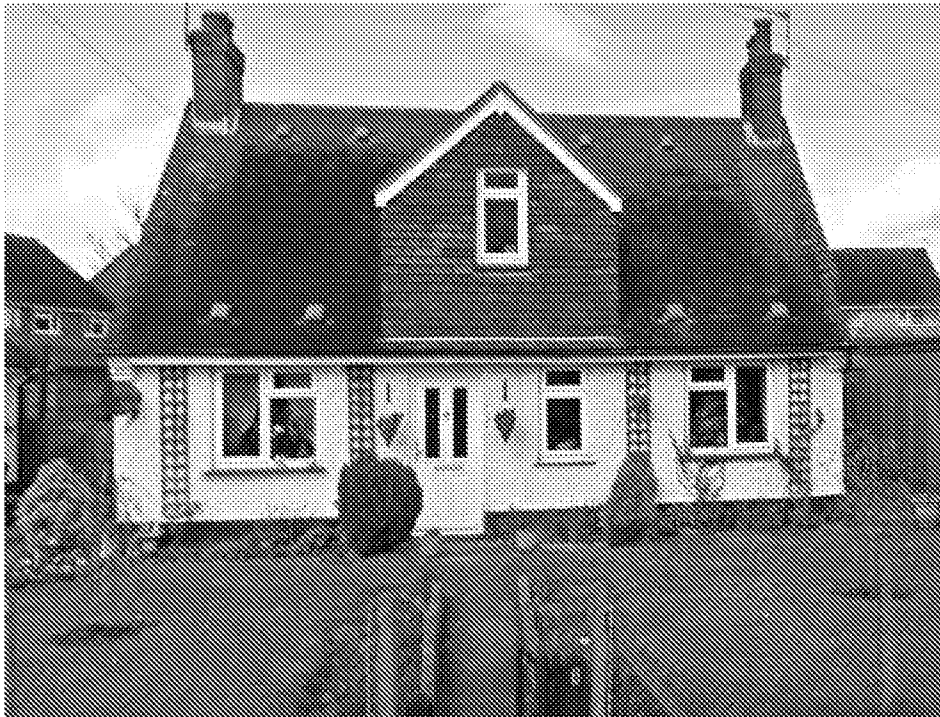
Chalet dwellings with feature gable forms and Chimneys
