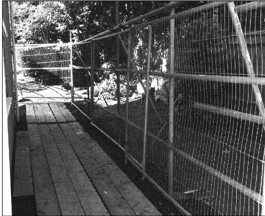
Scaffold board pedestrian ground protection
