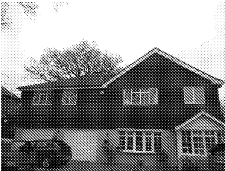
Photo 3: Building B3 (residential property, Oakdene, Hook Lane)
