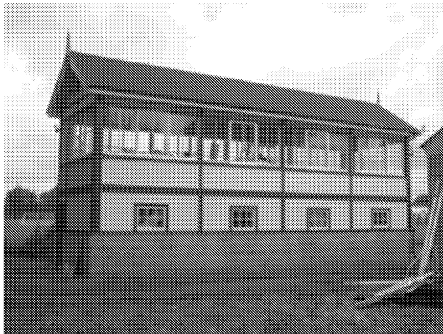
The adjacent Signal Box
