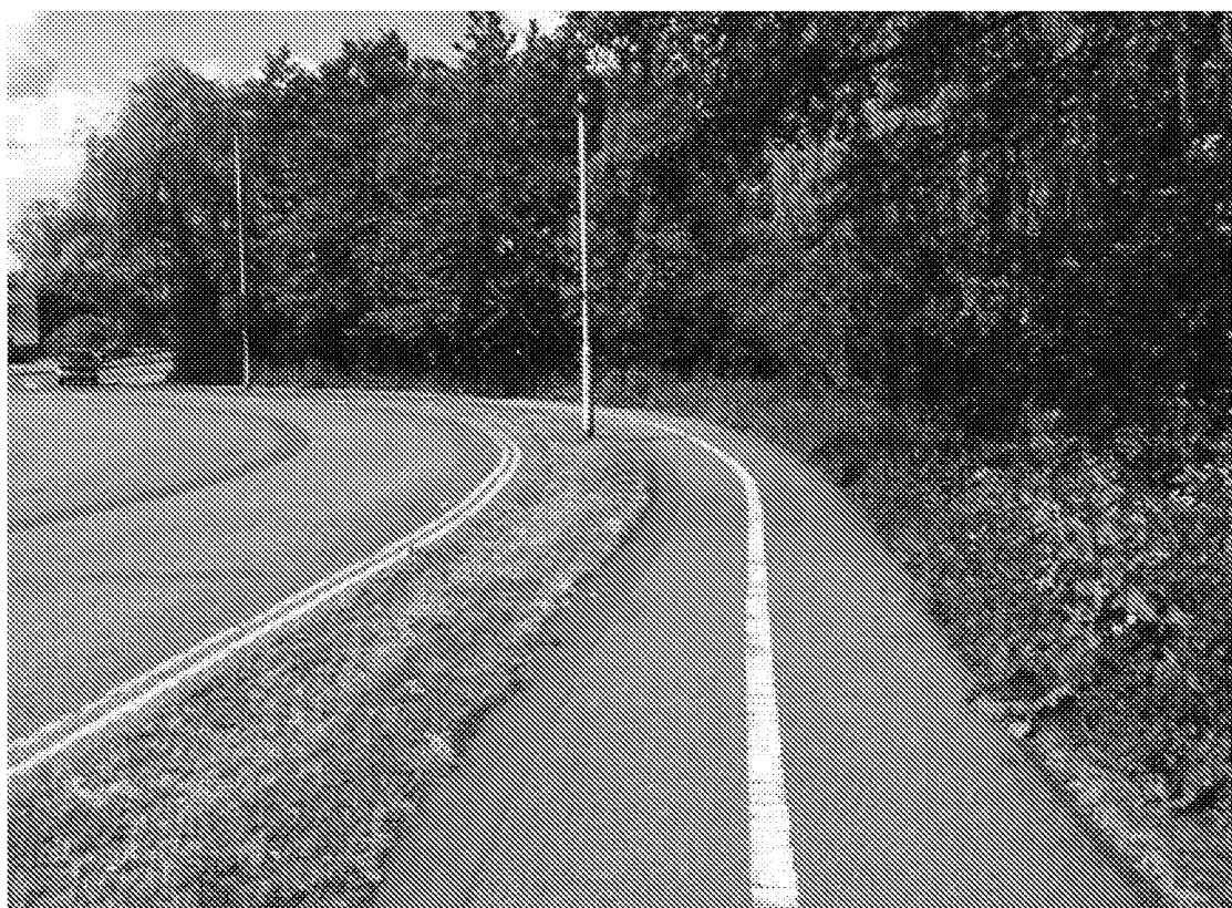
Figure 7.5 Substandard width on both sides due to segregation
