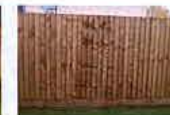
1.8M HIGH CLOSE BOARDED FENCING
