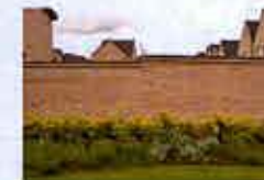
1.8M HIGH BRICK MASONRY WALL
