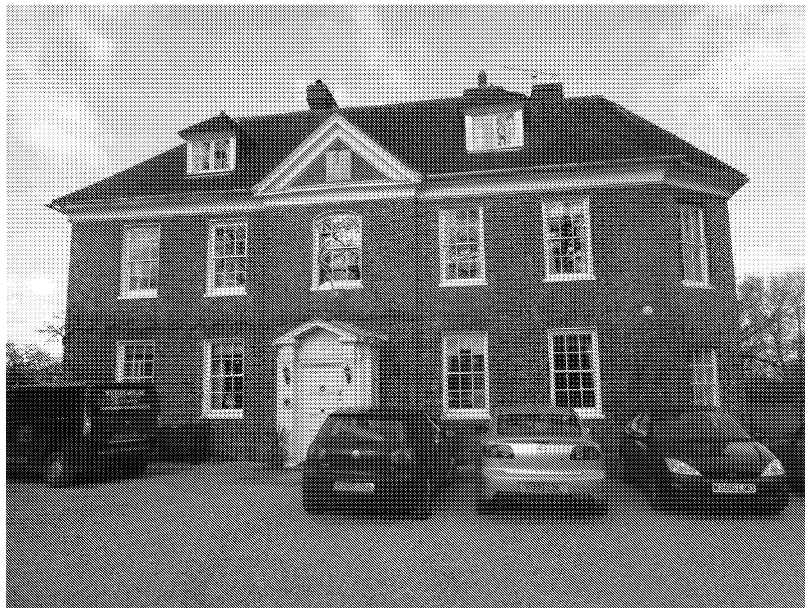
03: Main entrance of Nyton House (South Elevation)
