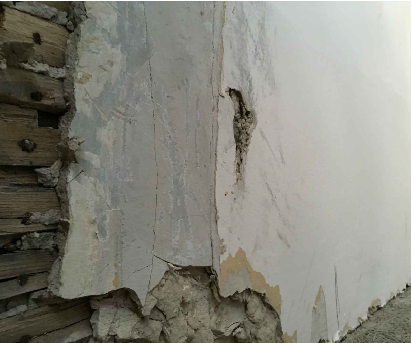
GENERALLY: LINING THROUGHOUT THE HOUSE
