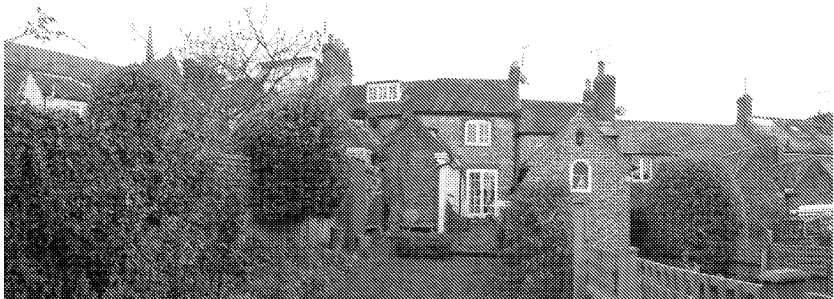
Panoramic rear elevation (no.37 to centre of picture)
