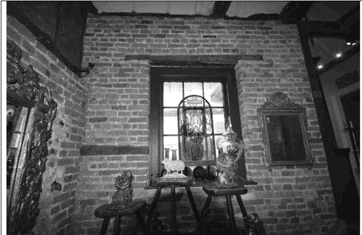
Plate 9: Northeast elevation of the stair turret with queen closers finishing the wall to accommodate a return and the corridor
