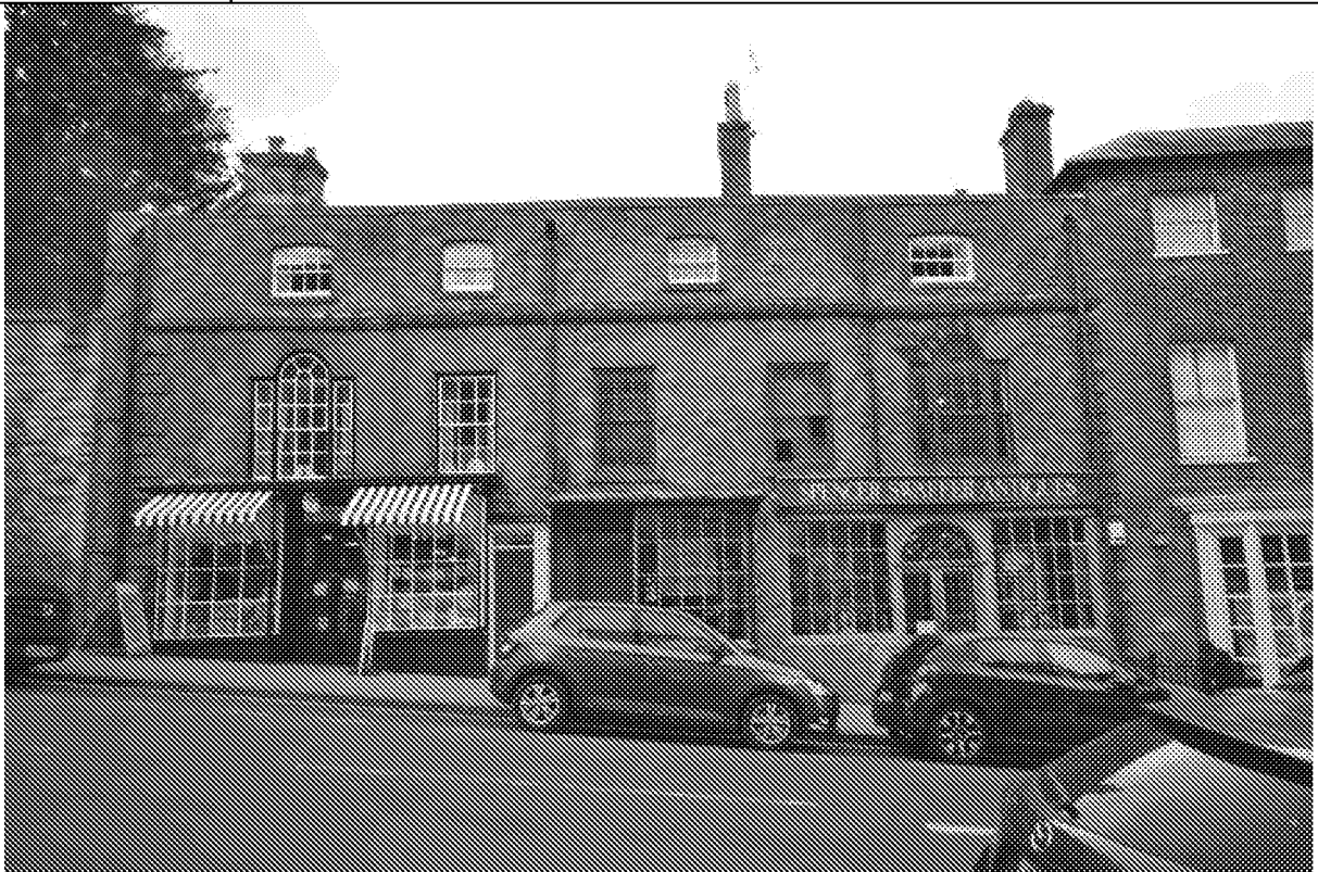
Plate 8: Mid 18th century frontage with late 18th and early 19th century shop fronts inserted
