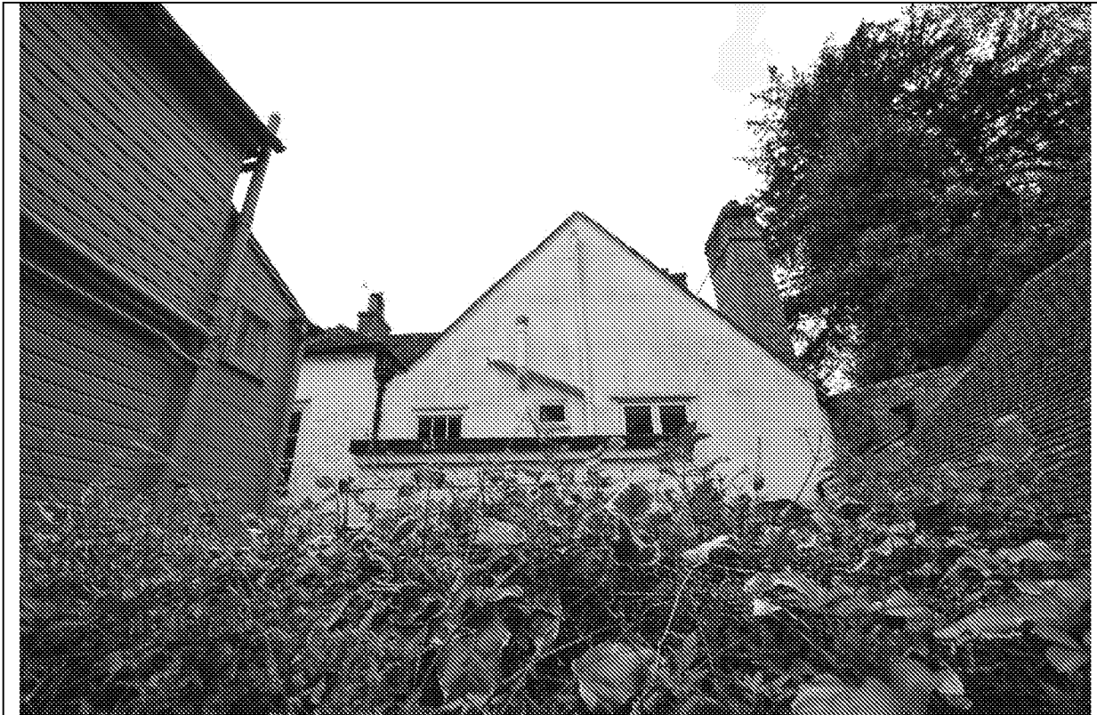
Plate 17: Rear of No. 34, under separate ownership
