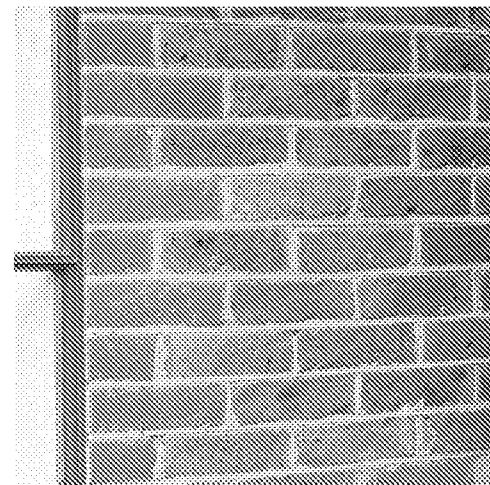
Face brickwork to match existing
