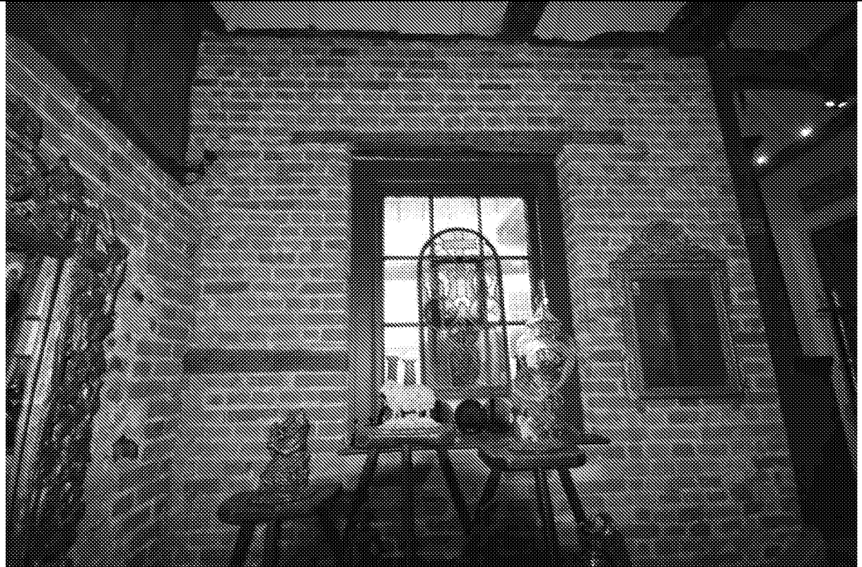
Plate 9: Northeast elevation of the stair turret with queen closers finishing the wall to accommodate a return and the corridor
