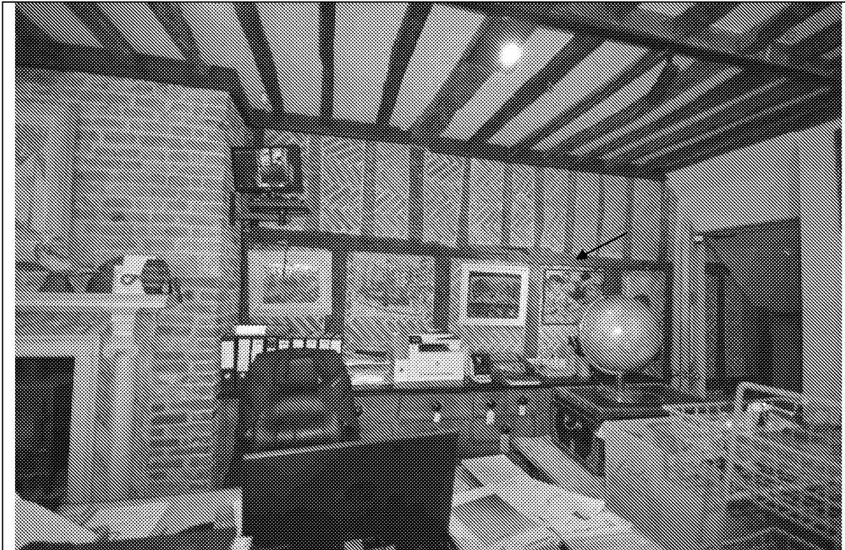
Plate 3: The early 17th century wall (wall-plate indicated by arrow)
