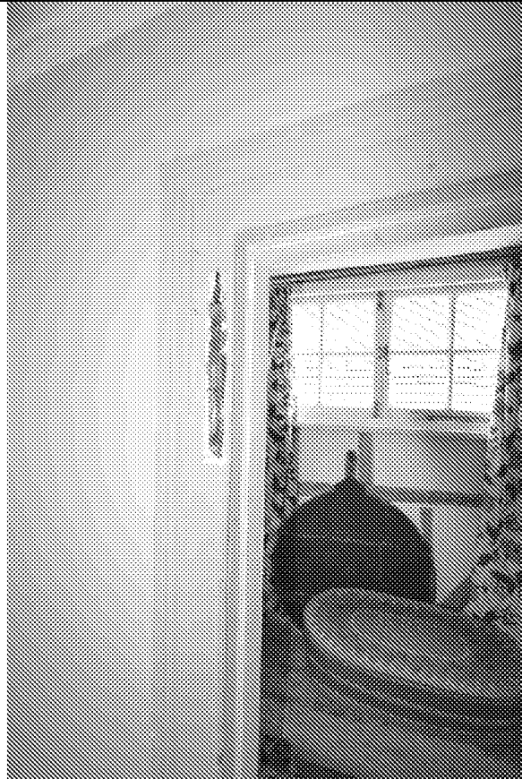
Plate 13: Georgian doorcase and scar for H-hinge in gallery 2, first floor of the late 18th century northwest extension
