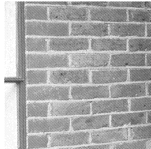
Face brickwork to match existing
