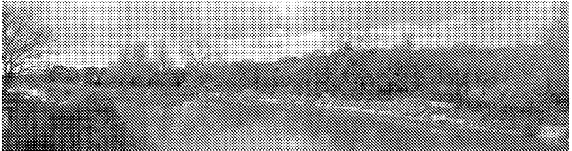
View from the A27 bridge over the River Arun looking south east towards the Site Photograph 17
