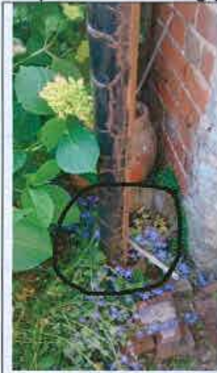
downpipe broken
