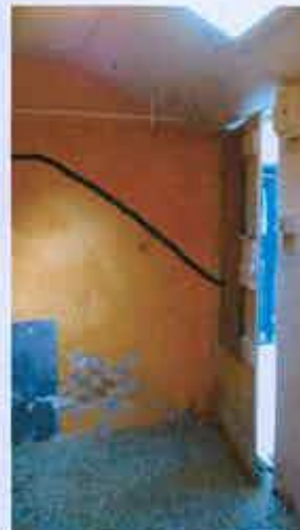
side wall by steps
